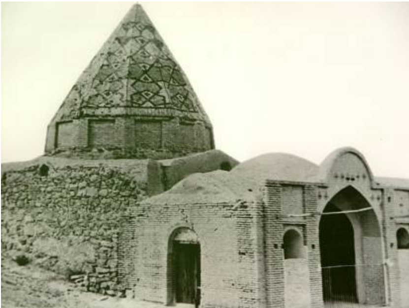
Figure 8.1: Zeinab Khatun Shrine: the southwestern side of the tetrapylon that its spans have been filled.
