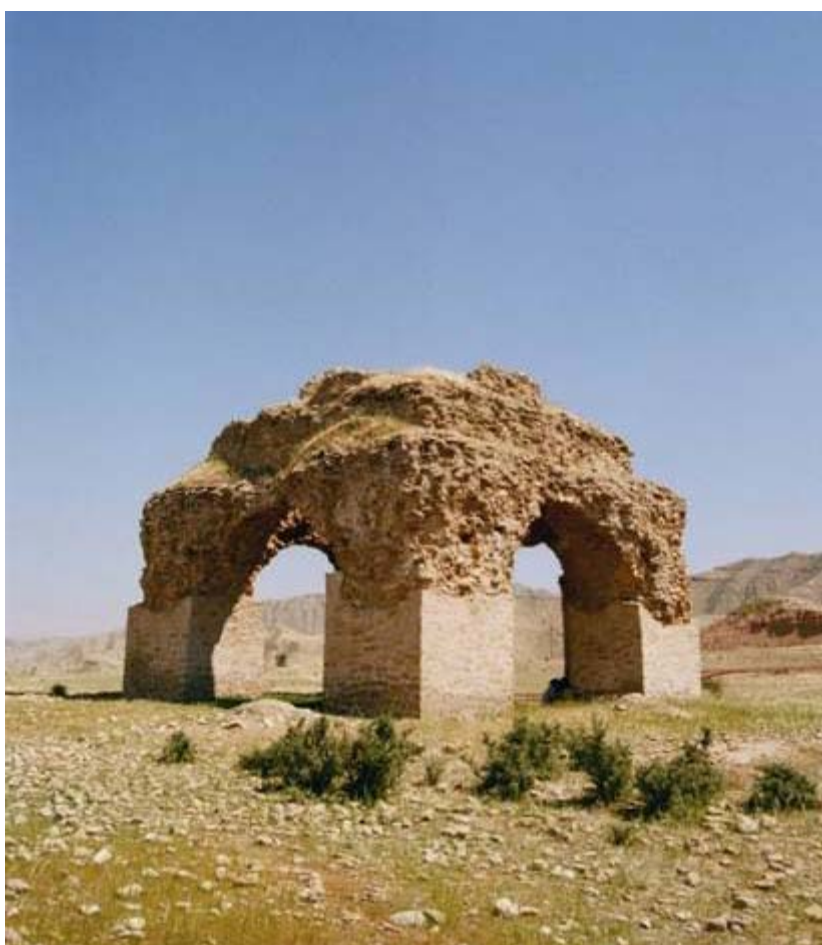
Figure 6.1: Kheyraabad Tetrapylon, the southwestern view
