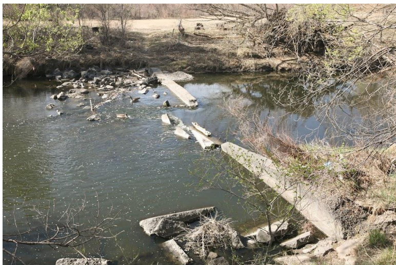
Failed concrete weir on Clear Creek
