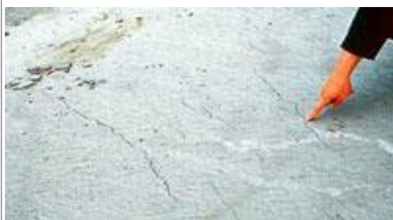
**(پلاستيکي انقباض) Plastic Shrinkage Cracking:**
