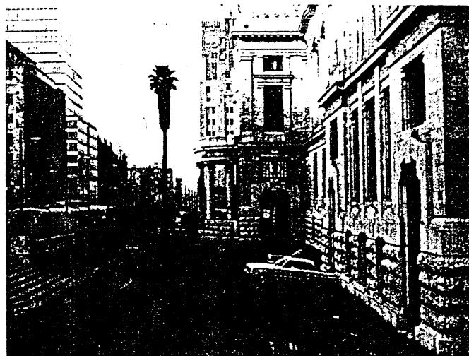
Fig. 1.3 Palacio de las Bellas Artes, Mexico City. The 2-m differential settlement between the street and the building on the right necessitated the steps which were added as the settlement occurred. The general subsidence of this part of the city is 7 m (photograph compliments of Raul Marsal).
