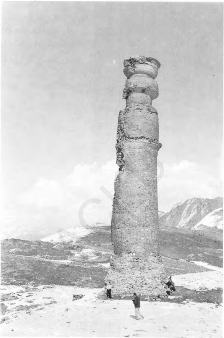
Illus. 4 in the 1980s the column was damaged by shelling
