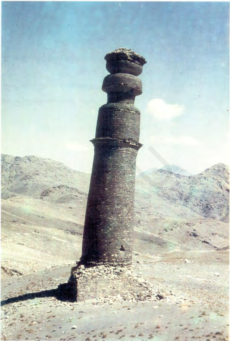
Illus. 1 the column tilted some 4 degrees to the south
