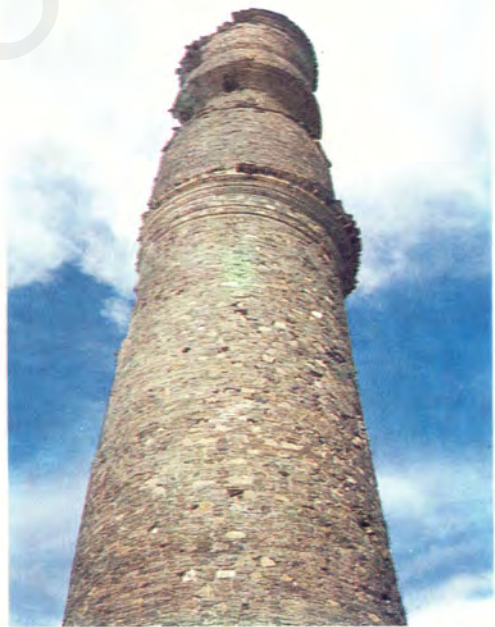
Illus. 6 the shaft was filled with rubble masonry
