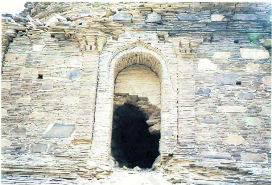
Illus. 7 Guldara Stupa: diaper masonry was a sophisticated building technique used by the Kushans
