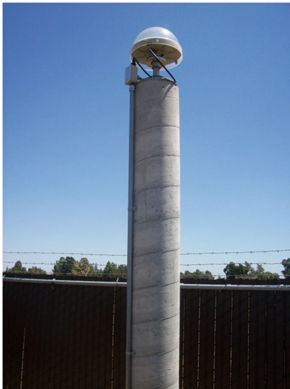
Fig. 6.1 GNSS CORS antenna on a monument pillar
