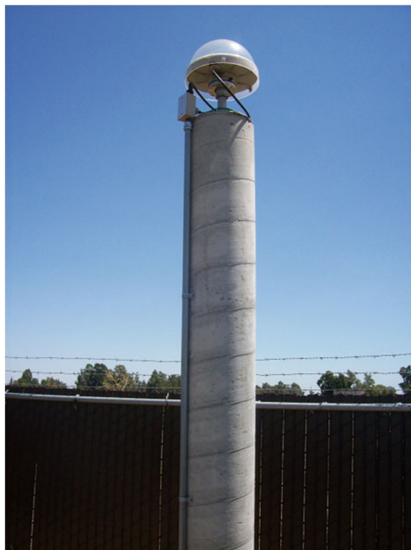
Fig. 6.1 GNSS CORS antenna on a monument pillar
