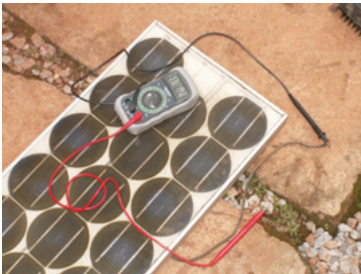
Figure 7.1: A solar panel
