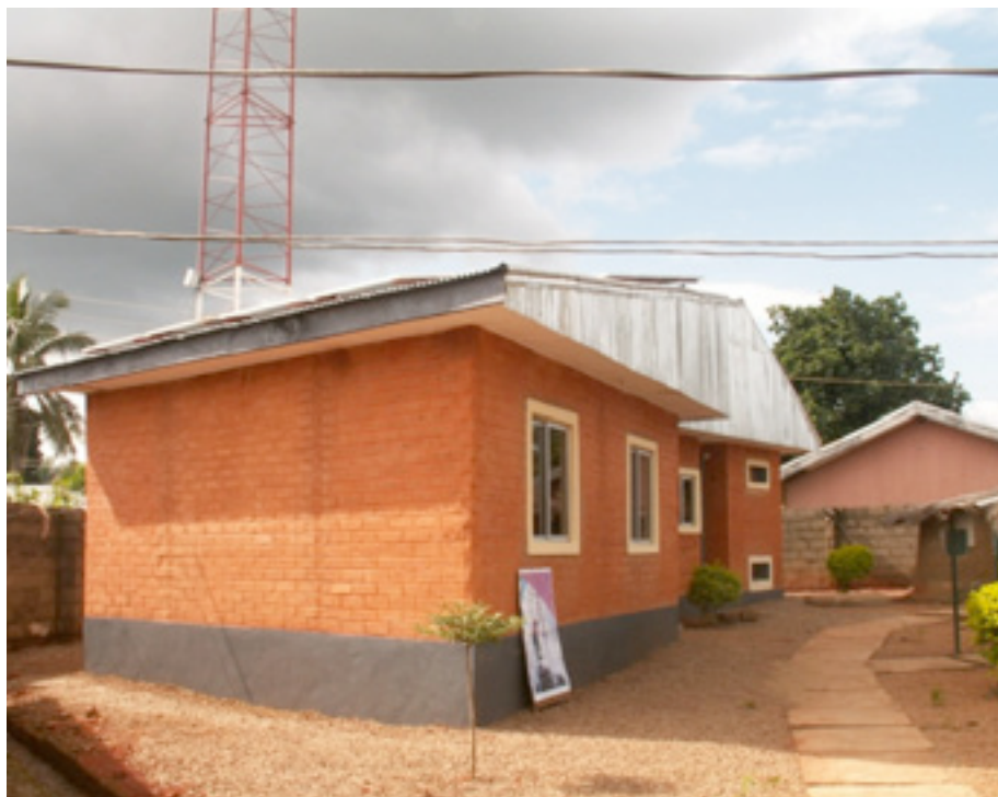
Figure 11.2: The NOC is built by locally made laterite brick stones, produced and laid by youths in Kafanchan.
