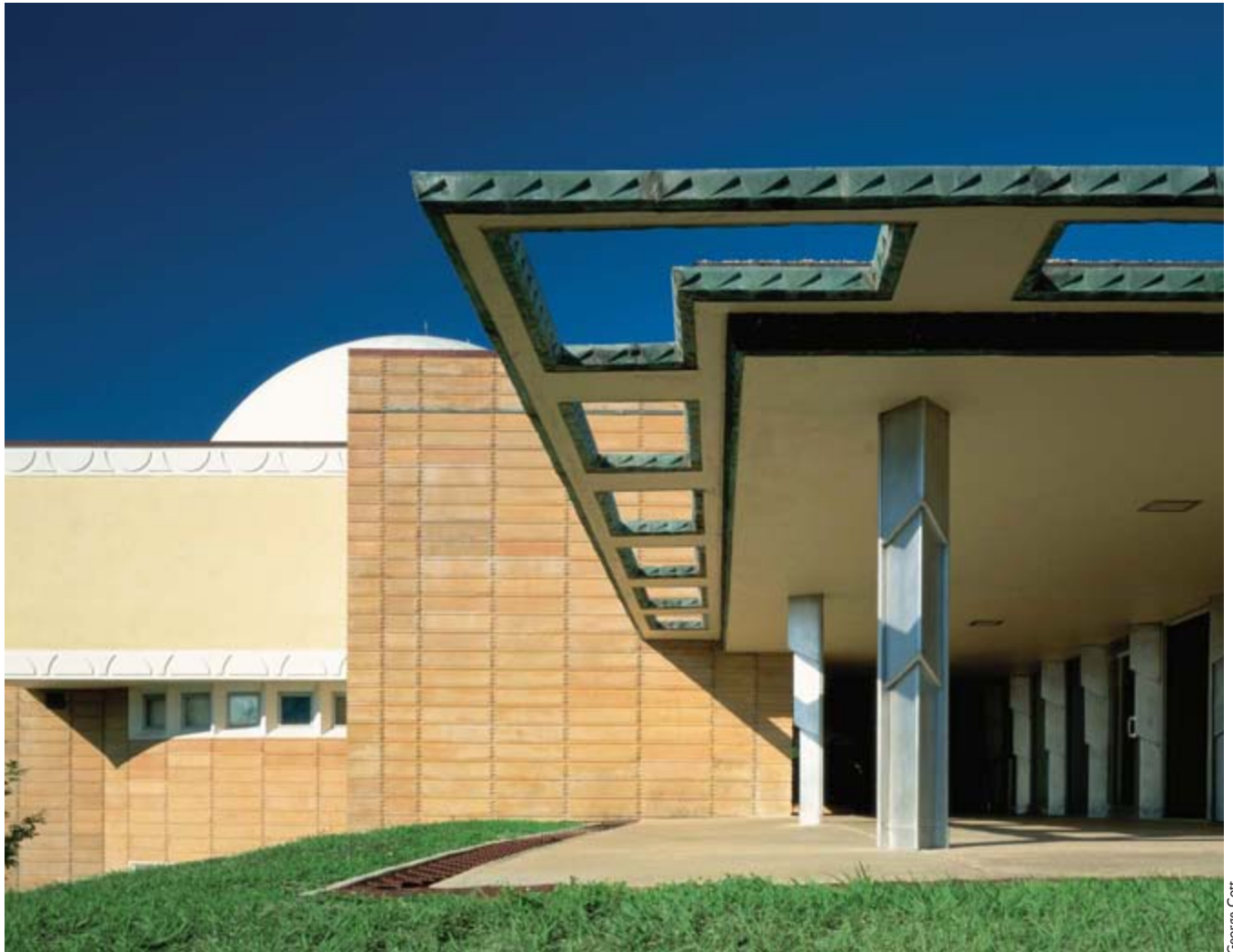
Original solar shading by Frank Lloyd Wright
