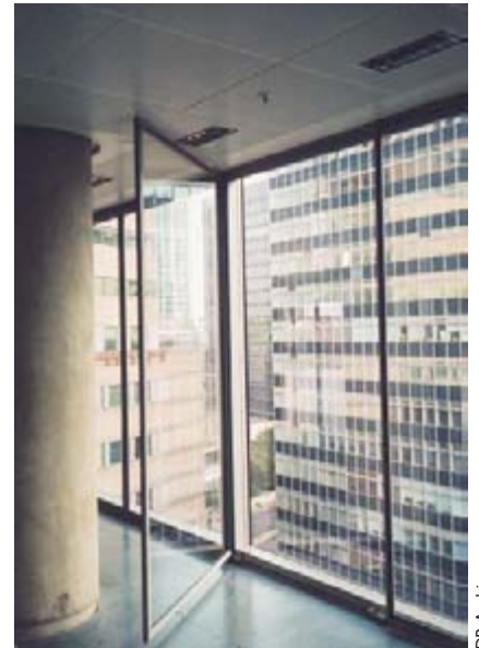
Detail of window with opening leaf
