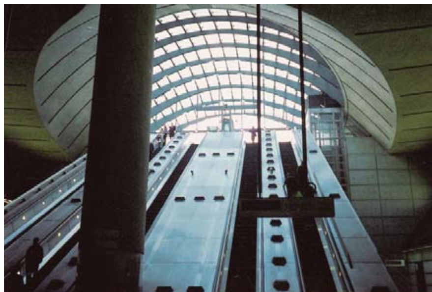
View up escalators to daylit canopy
