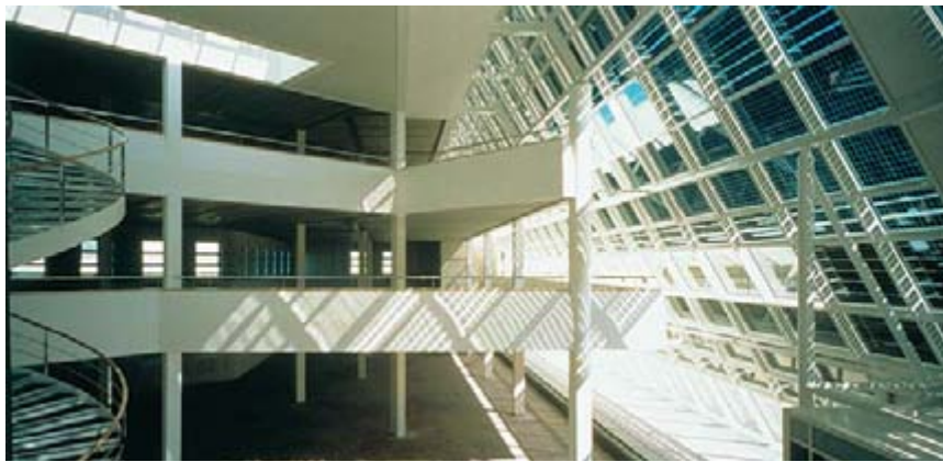
Solar Office, Doxford
