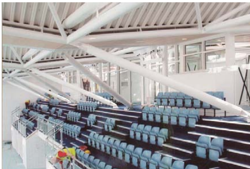
View of roof at seating level
