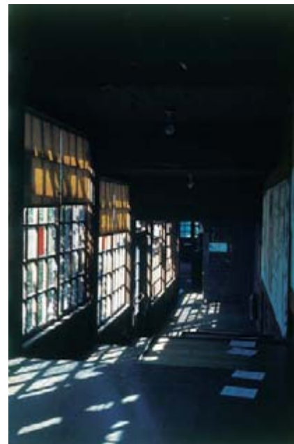
Staircase at Berkeley, USA. Shadow pattern conflict
