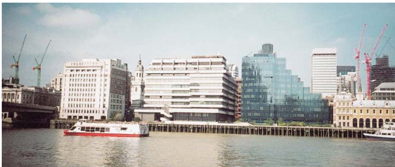
Three buildings on London's Embankment
