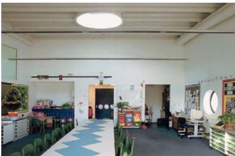
View of a classroom towards the rear, showing the effect of the daylighting and the circular rooflight.
