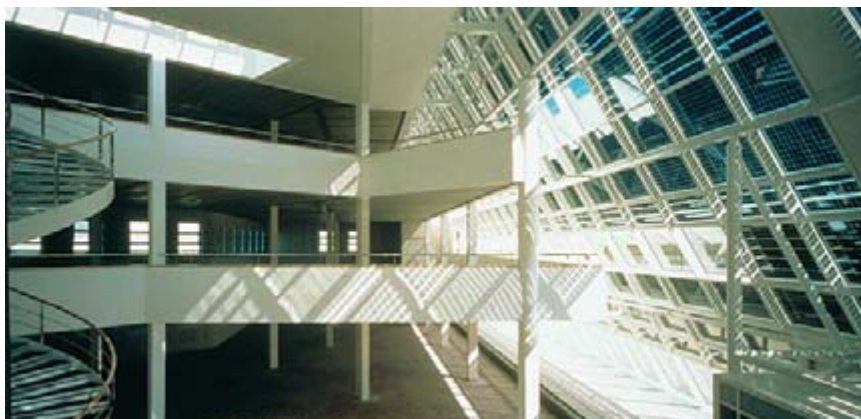
Solar Office, Doxford
