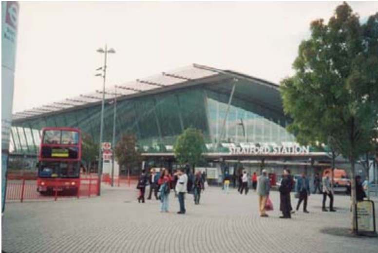
Exterior view to entrance
