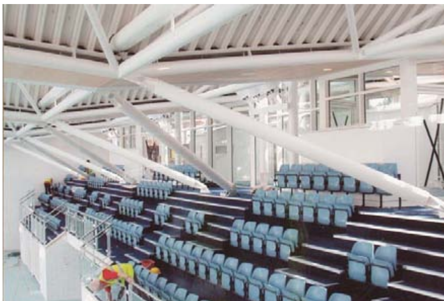
View of roof at seating level
