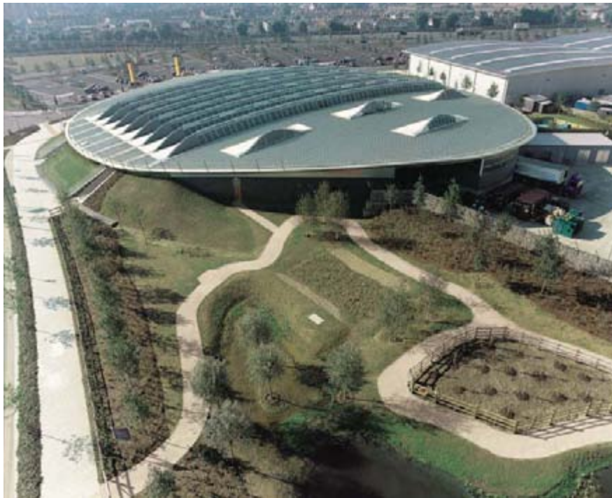
The roof from above
