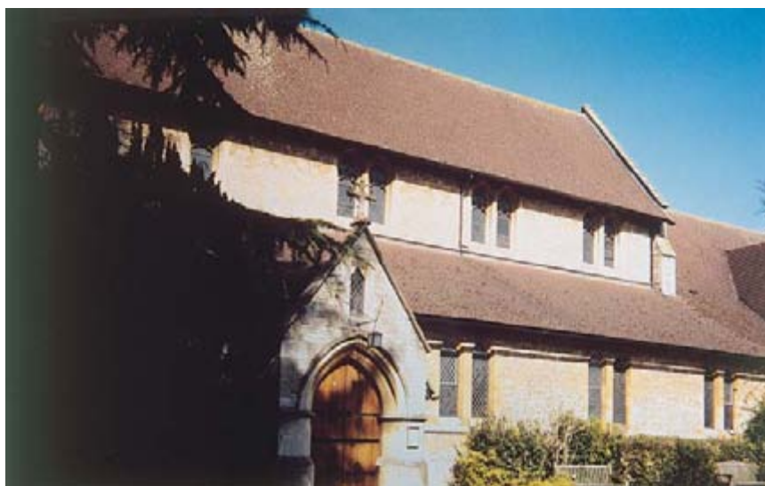
Extension to Boxmoor church
