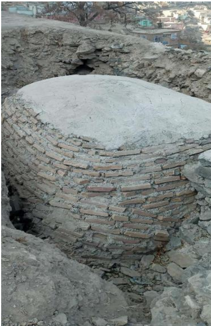
Guest room roof panorama (covering) of the Buddhist temple during renovation
