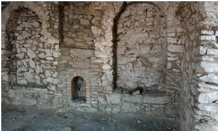
Interior pictures of the lower part of the Buddhist temple after renovation
