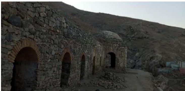
Front elevation Pictures of the Buddhist temple after renovation from the east
