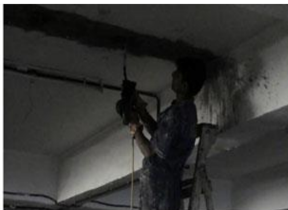
Figure 5. Epoxy injection in progress
