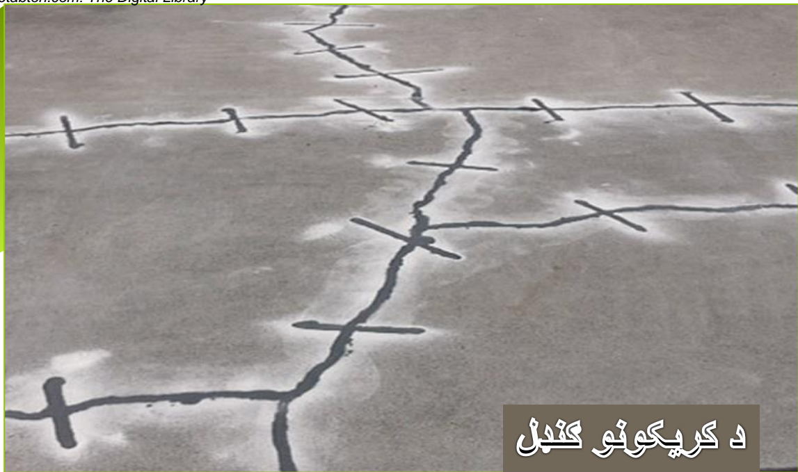
Figure 3: Stitching & Doweling
