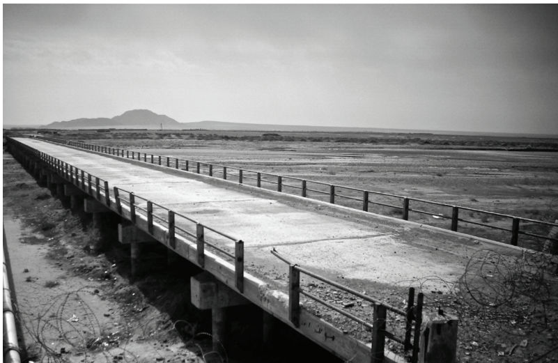
Arghestan Bridge, Kandahar province
