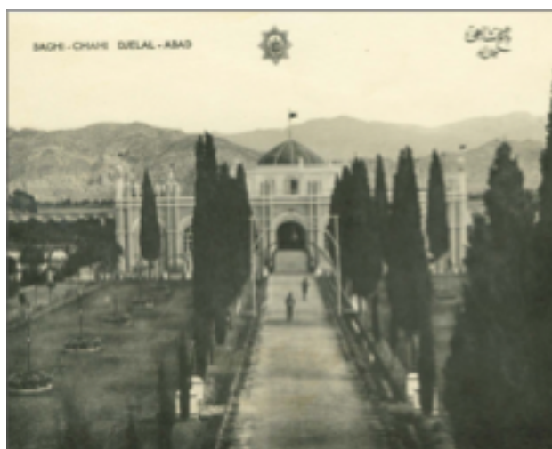
Figure 1 Nangarhar Palace, Photo from National Archive of Afghanistan
