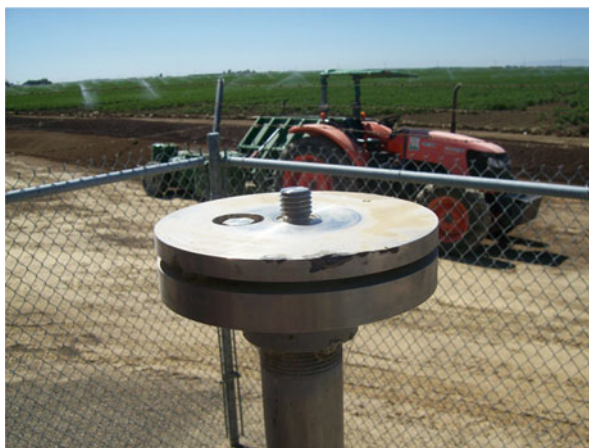
Fig. 6.4 Antenna mount without a GNSS antenna
