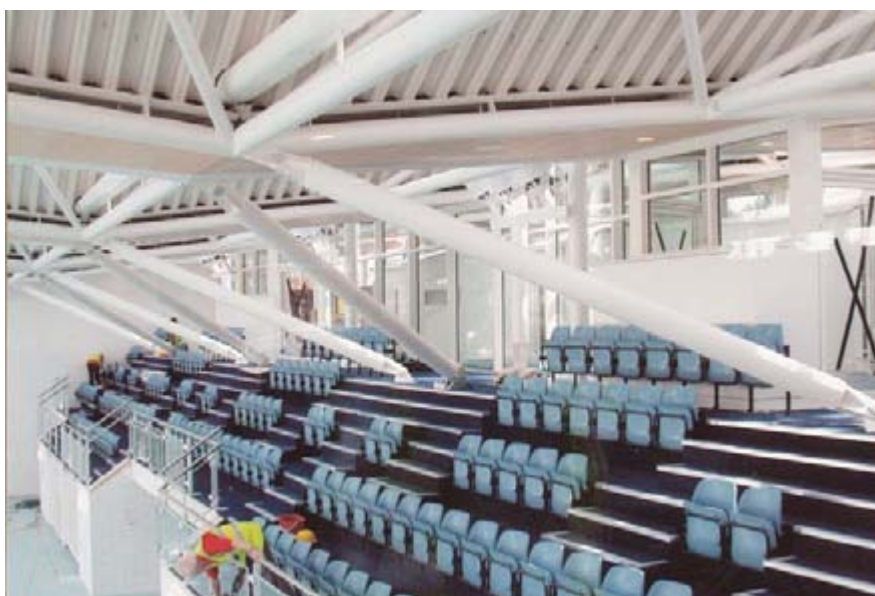
View of roof at seating level
