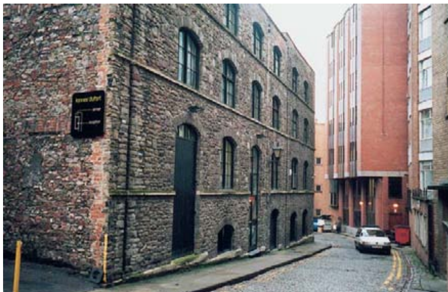
The exterior of the building
