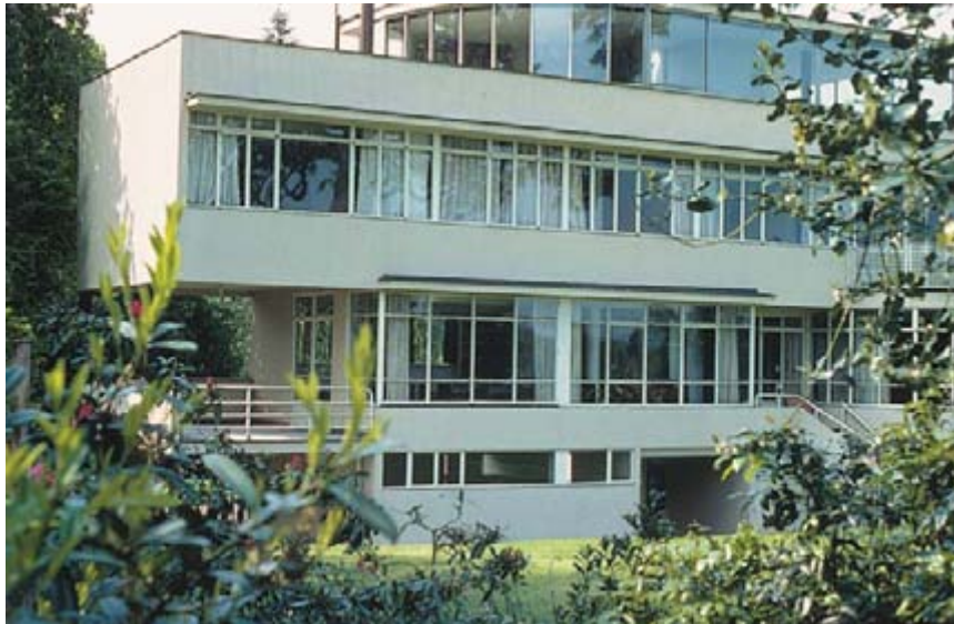
Connell Ward and Lucas House, Moor Park
