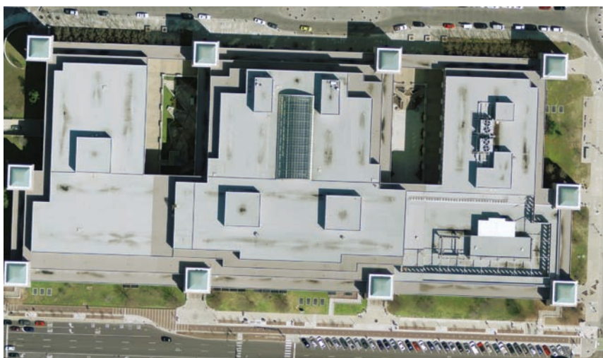
FIGURE 17.1 Building with step edges on its roof.
