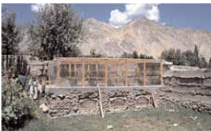
Figure 29: A type of solar dryer, made with mud walls.
