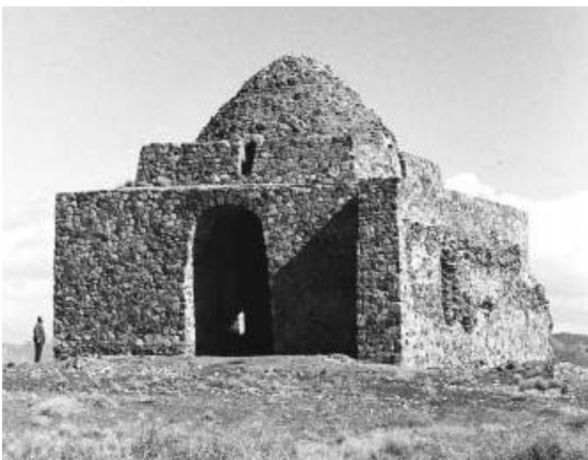
Figure 11.9 and 11.10: Bazeh-e Hur Tetrapylon, Neyshabur: the tetrapylon is located on the left side of the Neyshabour road to Torbat-e Heydariieh, after the village of Robat Sefid.
