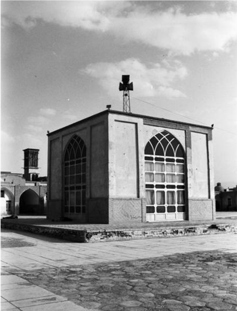
Figure 11.8: Mosalla Tetrapylon, Yazd
