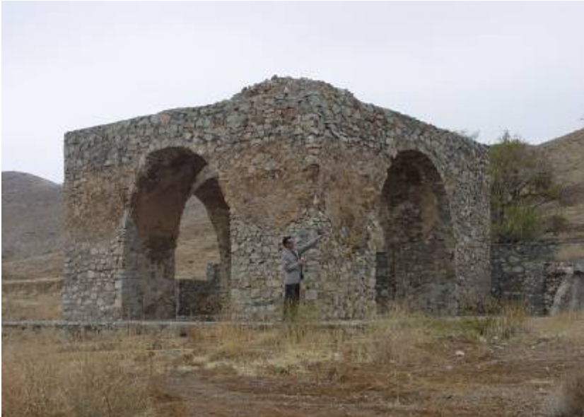
Figure 5.2: Nevis Tetrapylon, the western view
