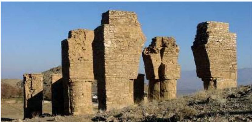
Figure 4.6: Botkhaneh Tetrapylon, the northern view
