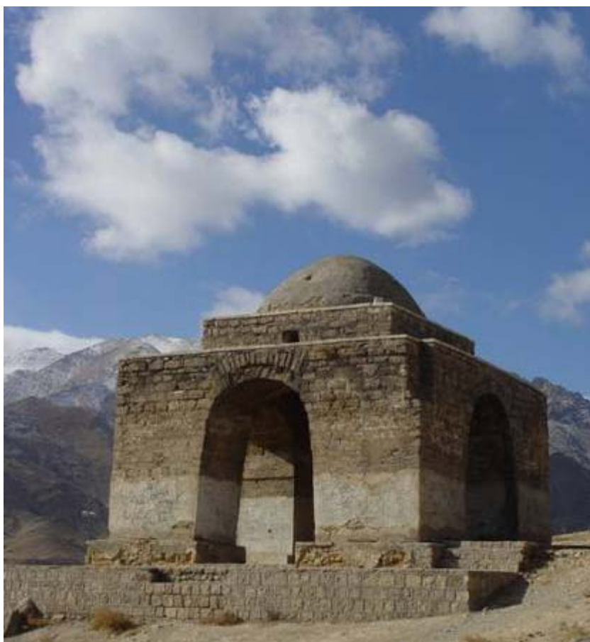
Figure 3.1: Niasar Tetrapylon, the western view
