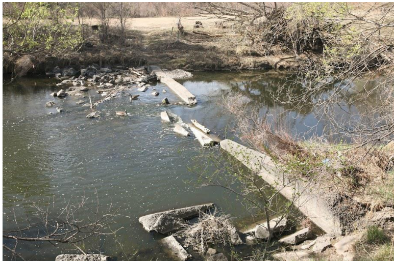
Failed concrete weir on Clear Creek
