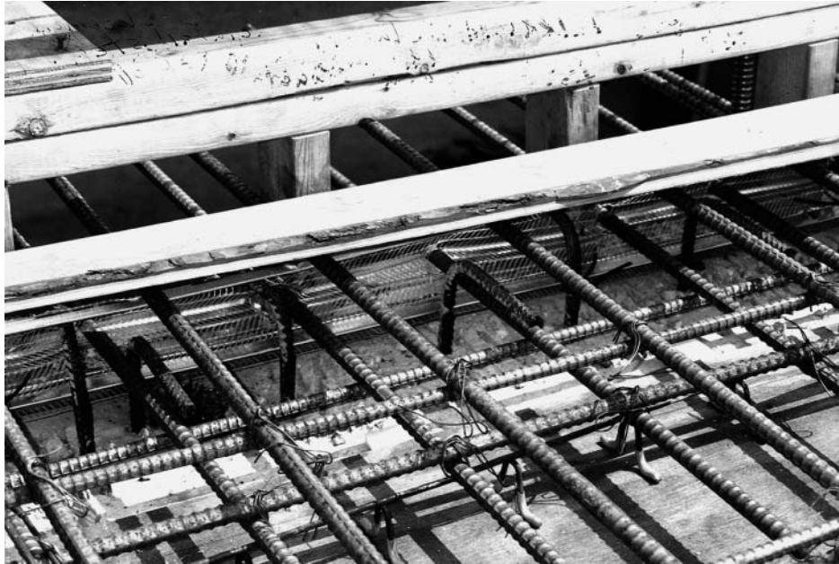
Reinforcing bars. Note the supporting metal chairs.
