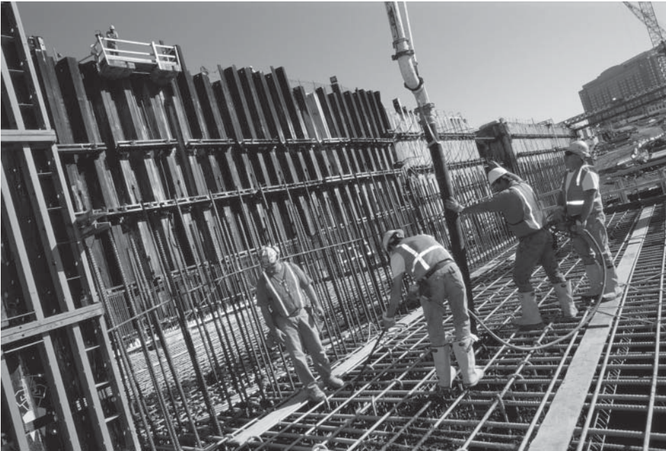
Pouring concrete, Big Dig, Boston, Massachusetts.
