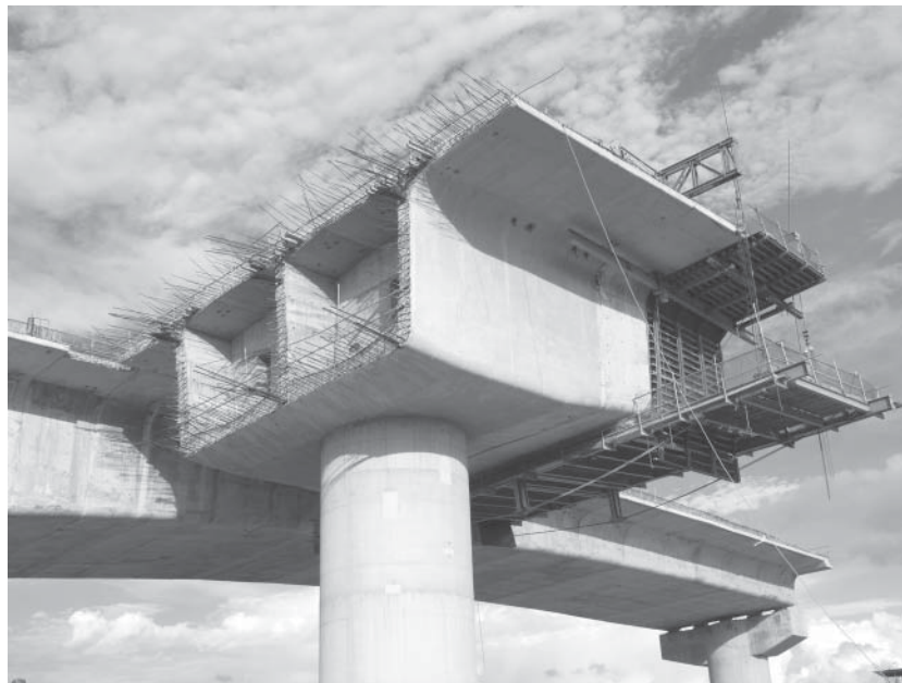
Segmental prestressed concrete bridge construction.
