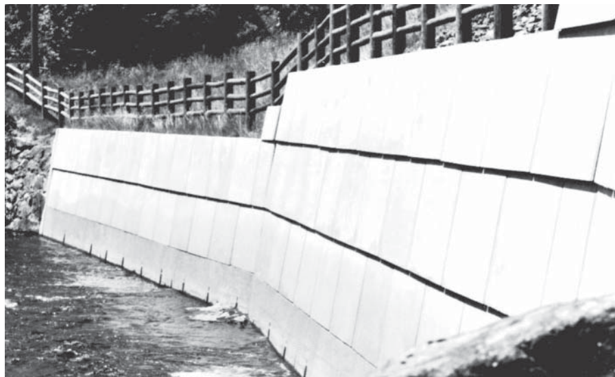
Retaining wall for United States Army Corps of Engineers, Colchester, Connecticut. Constructed with precast interlocking reinforced concrete modules.
