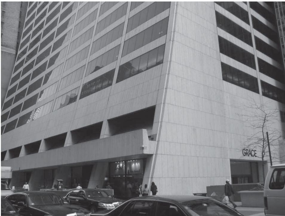
Buttress shear wall, New York Hilton, New York, New York.
