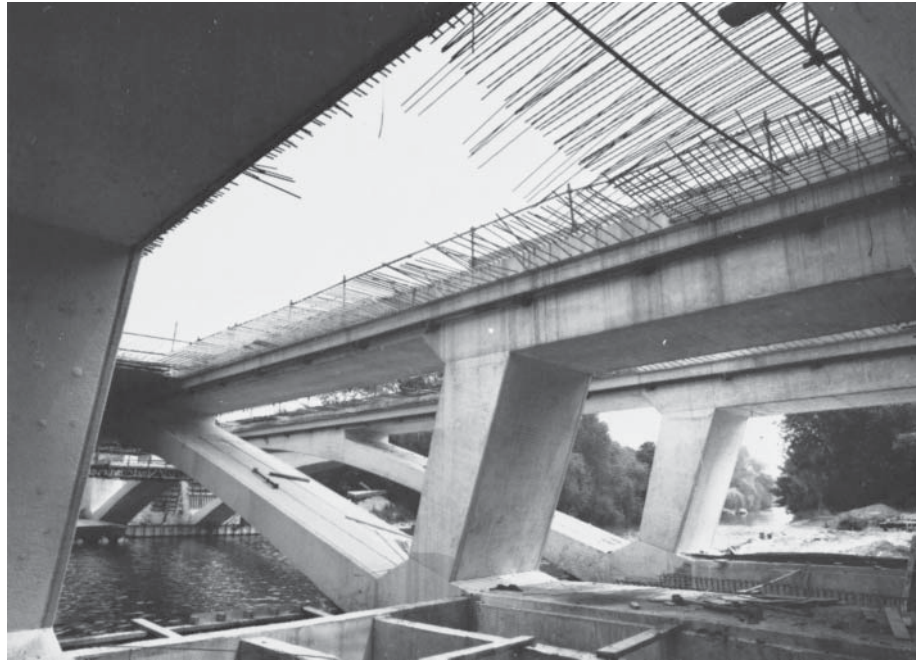
Prestressed concrete Runnymede Bridge over Thames River near Egham, Surrey, England.
