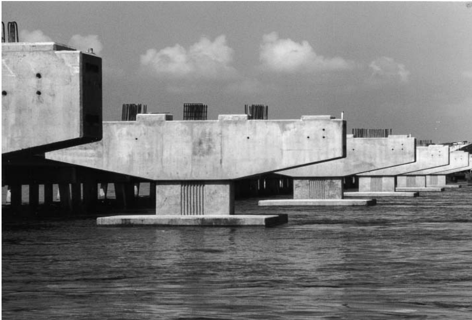
Columns and hammerhead cap forms for the Gandy Bridge, Tampa, Florida.
