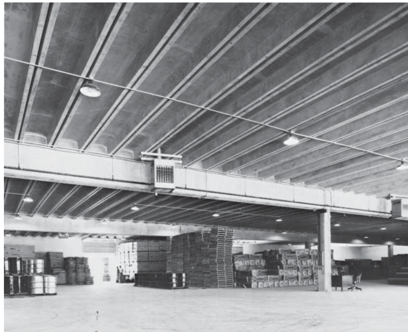
Prestressed concrete channels, John A. Denies Son Company Warehouse #4, Memphis, Tennessee.
