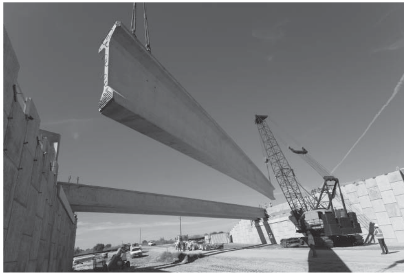
Prestressed bridge girders during erection.
