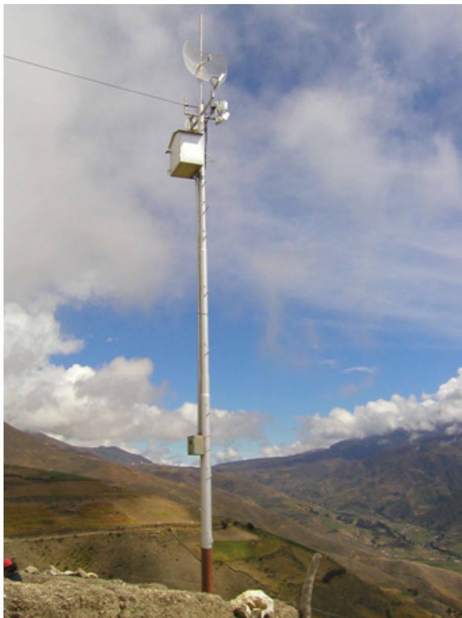
Figure 8.3: A simple self-supporting tower.
