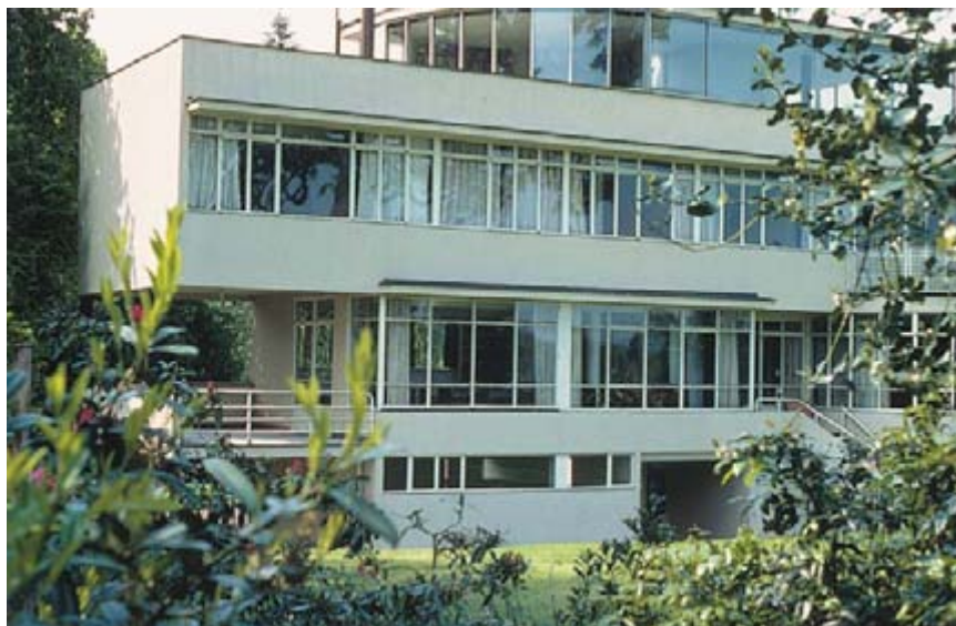
Connell Ward and Lucas House, Moor Park
