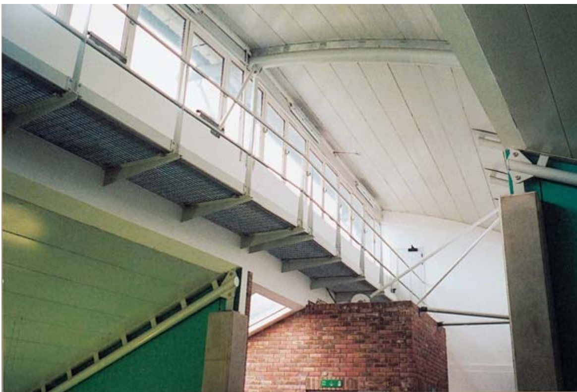
Clerestory glazing at high level with catwalk for maintenance
