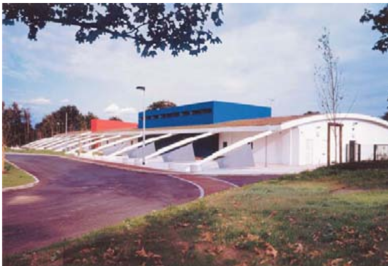
View of the school from the south, classroom side
