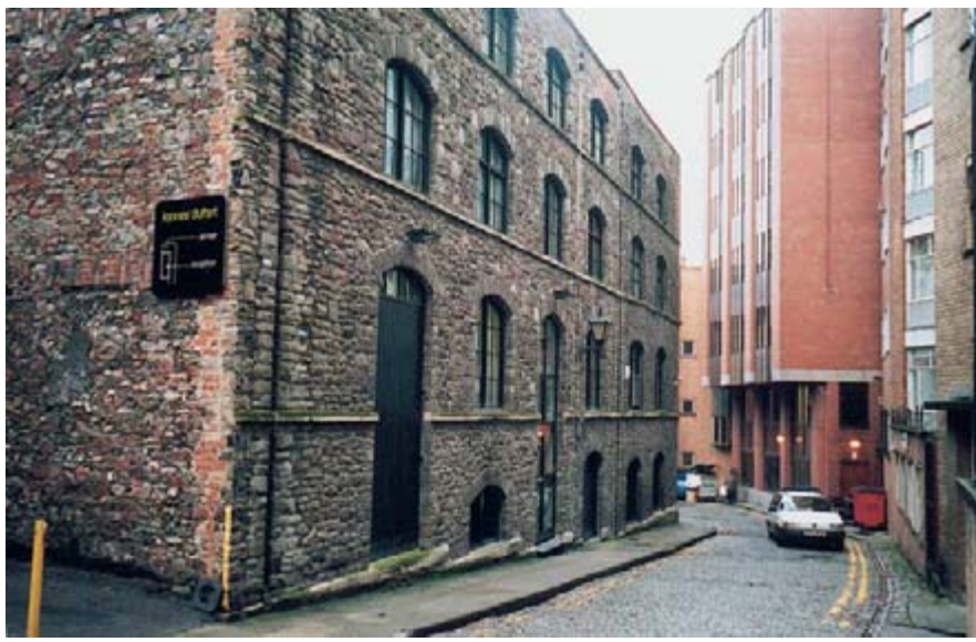
The exterior of the building
