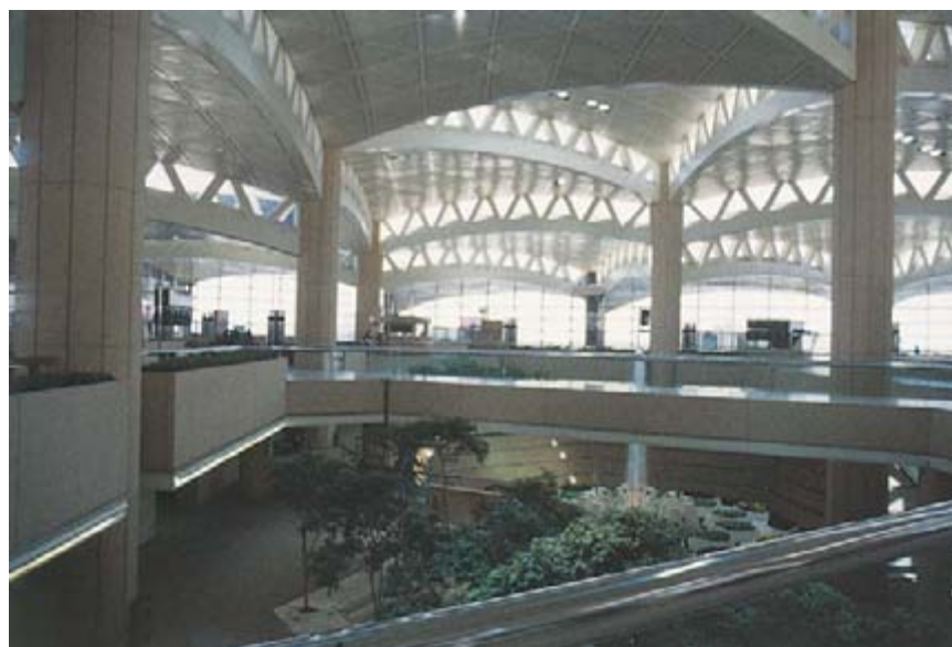
The King Khalid Airport, Riyadh, Saudi Arabia
