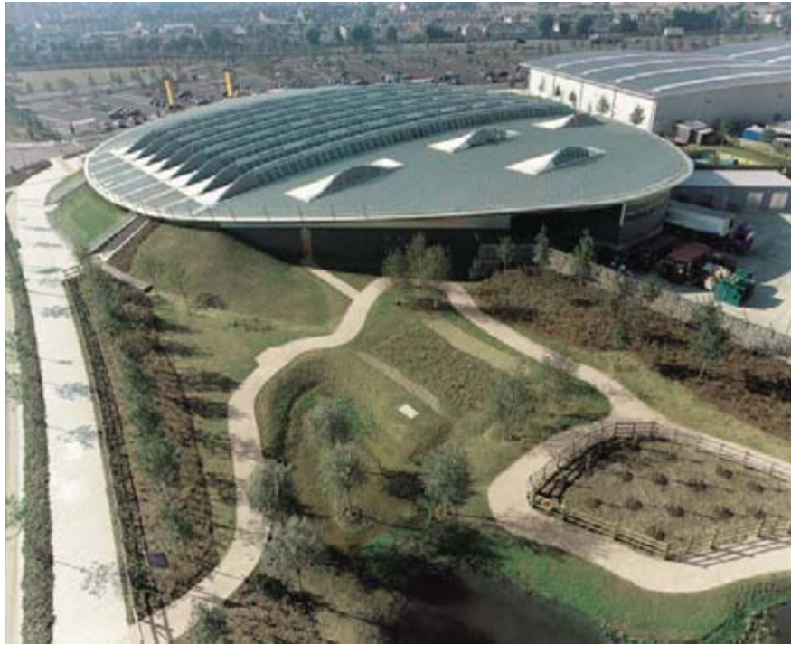
The roof from above
