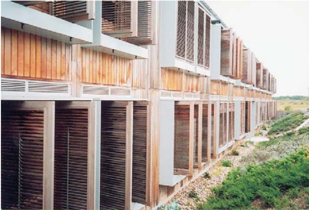
External hand-operated louvres to the south east elevation, for the occupants close to the windows
