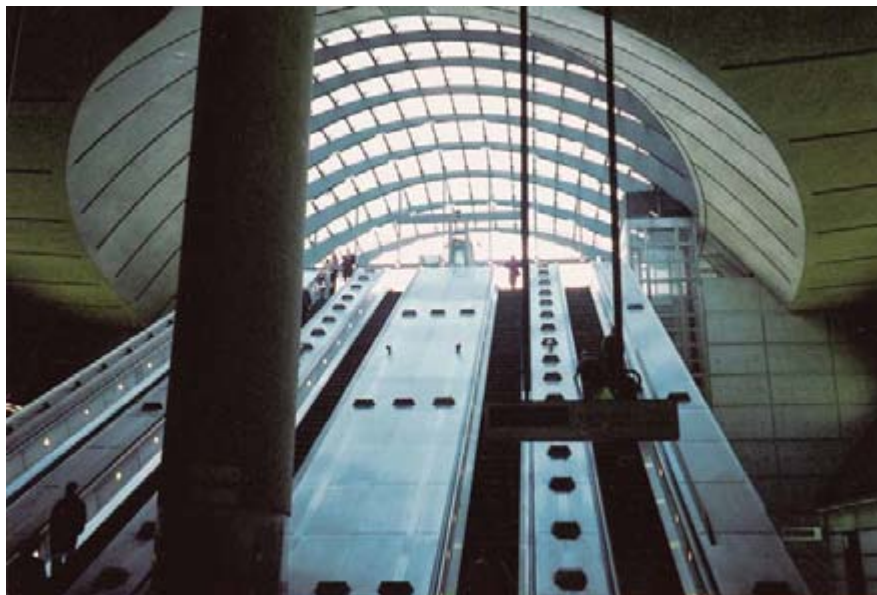
View up escalators to daylit canopy
