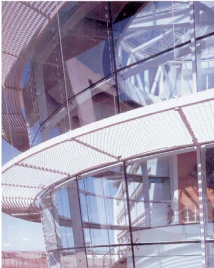
Window detail to show sun control
