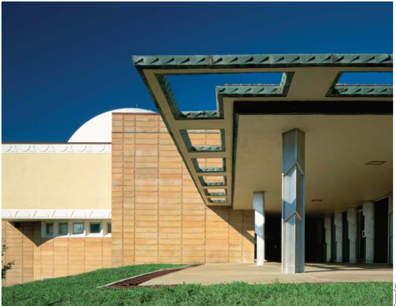
Original solar shading by Frank Lloyd Wright
