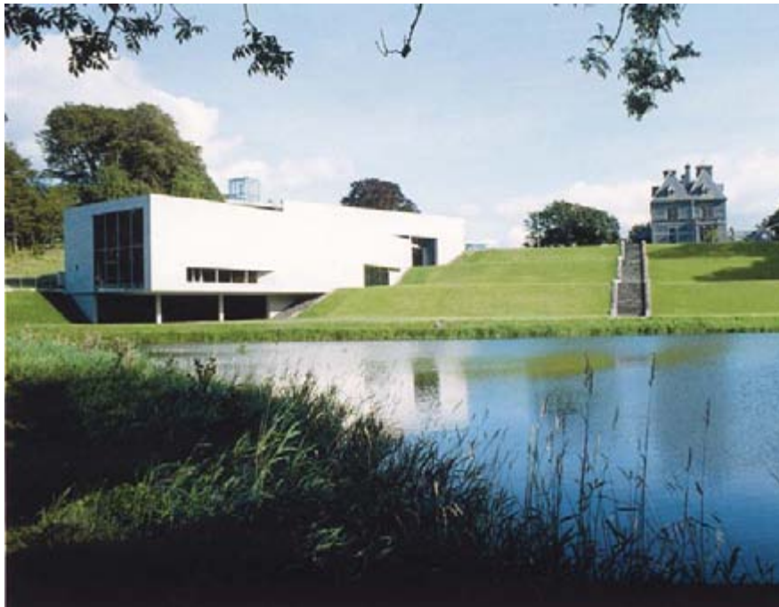
Exterior of the building
