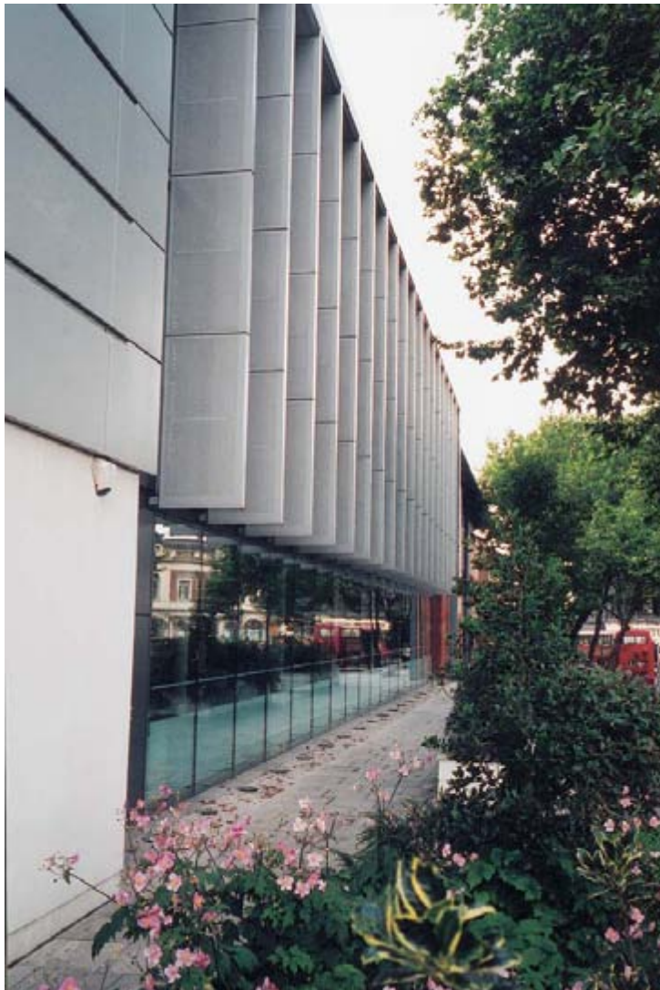
Exterior view during the day showing the fins
