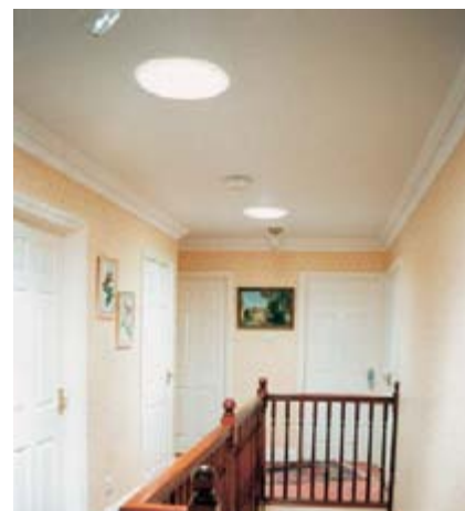
Photograph of typical light-pipe installation seen from inside the building
