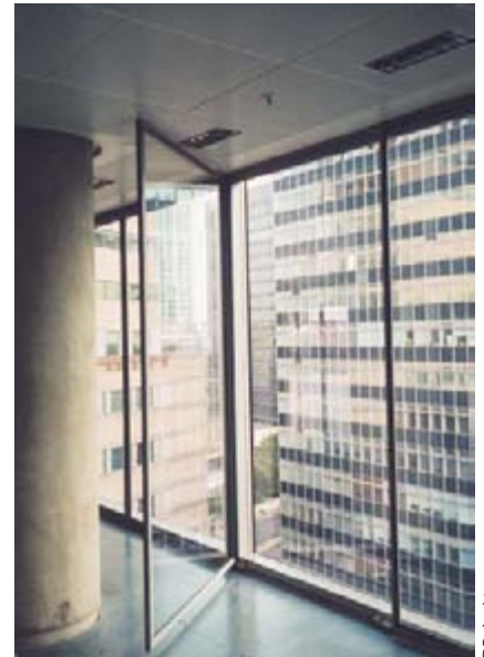
Detail of window with opening leaf
