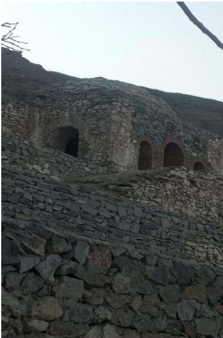
Front elevation Pictures of the Buddhist temple after renovation from the north
