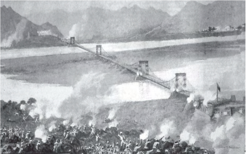
Chakdara Bridge Under Attack.
