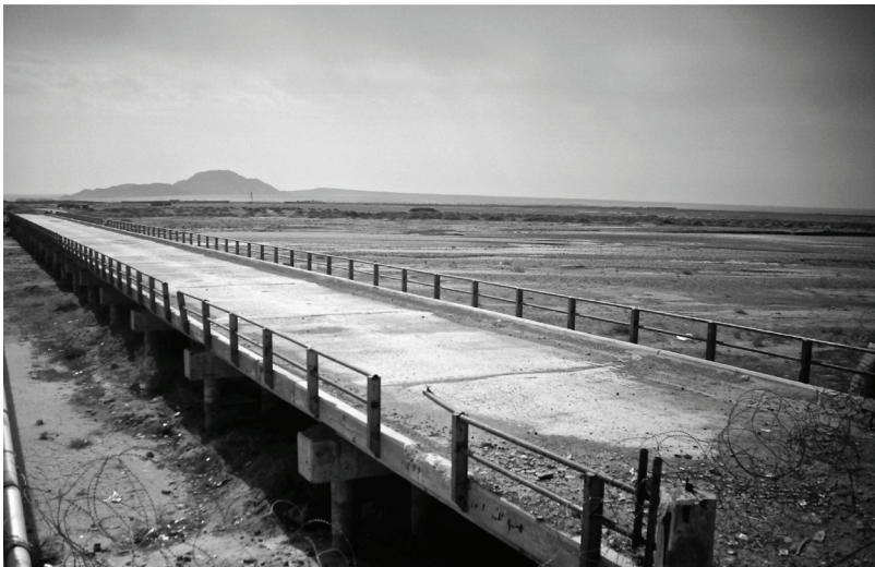
Arghestan Bridge, Kandahar province
